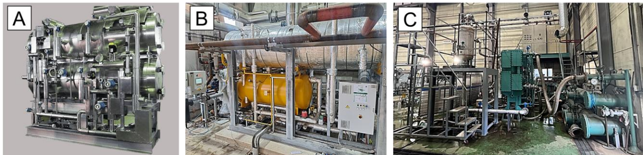
Figure 8: (A) This BS Nova H 2 O/LiBr AHT demonstrator at Tüpraş (Turkey), developed in the EU Horizon 2020 Indus3Es project (200 kW; heat upgrade 95 → 135 °C; COP 0.50) (Indus3Es, 2018). (B) BS Nova H 2 O/LiBr AHT demonstrator at paper mill in Cuartiere di Guarcino (Italy) developed in the EU Horizon Push2Heat project (715 kW waste heat at 85–90 °C upgraded to 340 kW steam at 3.3 bar(a), 126 °C, 0.6 t/h; COP 0.48), coupled with a thermocompressor to produce 6.5 bar(a), 162 °C steam (2.4 t/h) using 14.5 bar motive steam (1.8 t/h) (Alonso et al., 2025; Push2Heat, 2025, 2022) (C) H 2 O/LiBr AHT system developed by World E&C (260 kW; absorber temperatures 118–124 °C; heat source 89–82 °C; heat rejection 24–32 °C (Arpagaus et al., 2026b).
